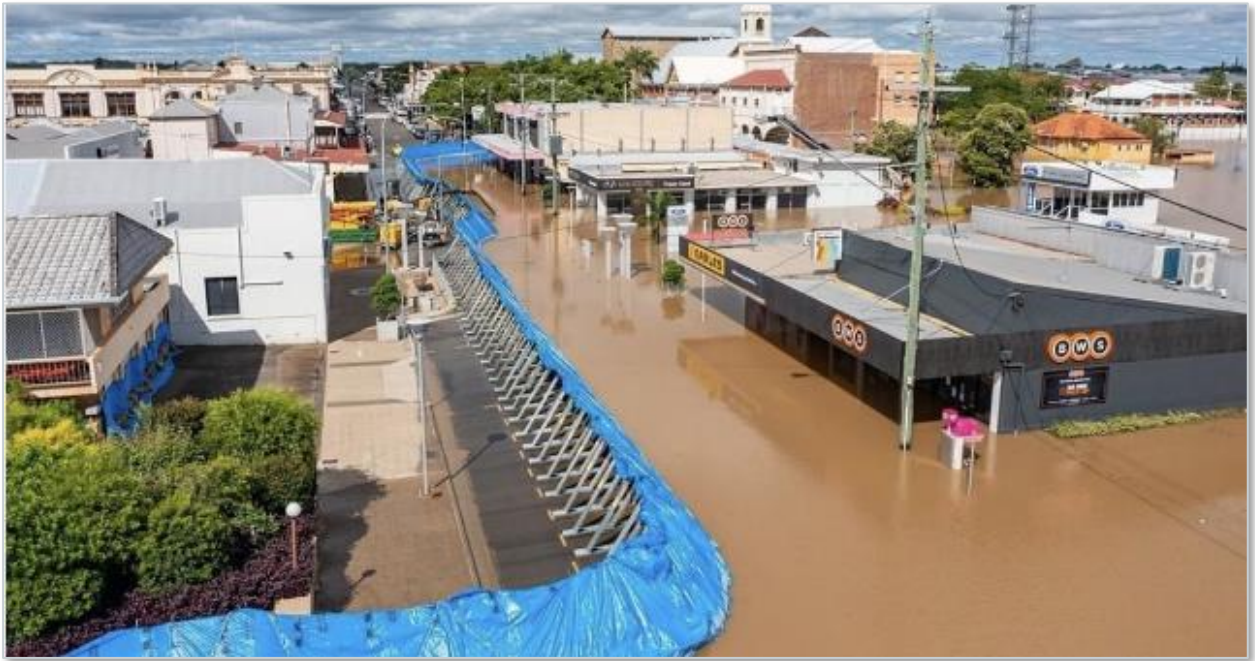
Figure 29 - Inflatable temporary flood barrier
