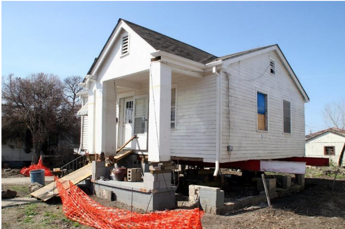
Figure 25 House being raised in New Orleans
