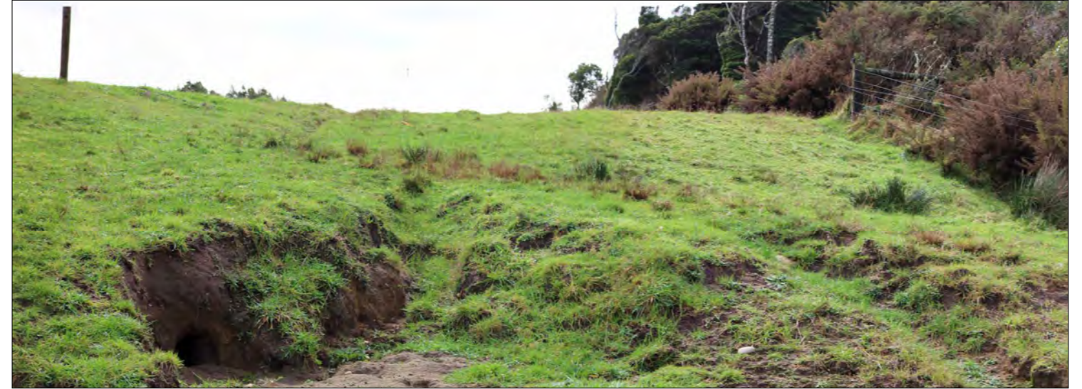
2. Erosion and slumping evident within Application Area.
