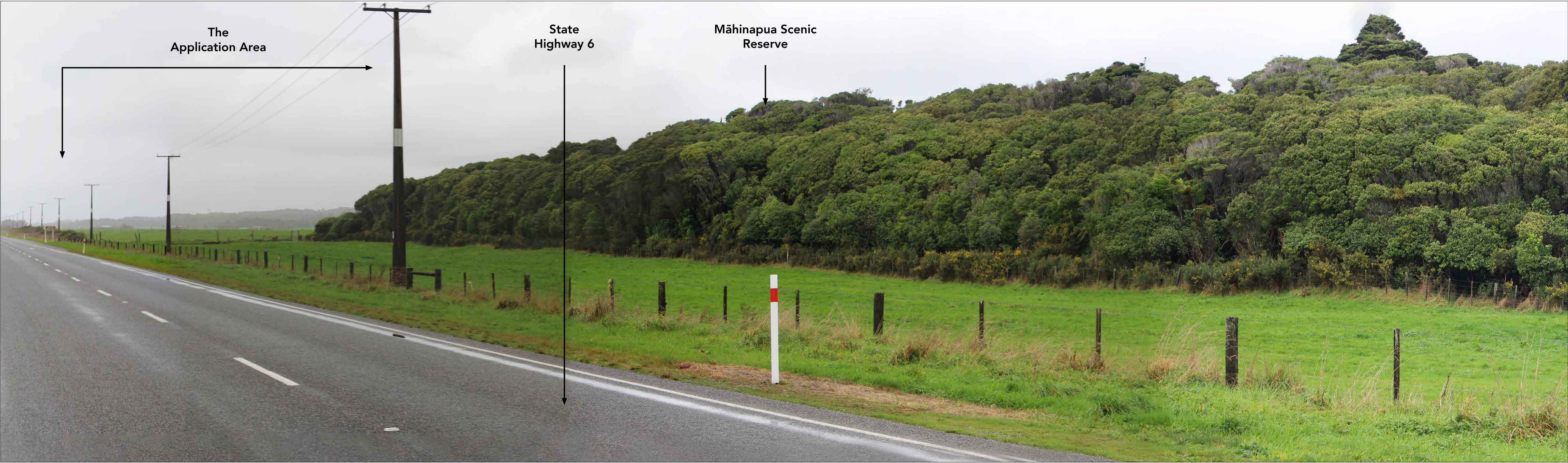
Viewpoint 1: Panoramic view taken beside the driveway of 866 Ruatapu Road (SH6). This viewpoint is looking in north along SH6 towards the Application Area. Taken on the 31st May 2023 with a Canon 600D camera with a 50mm lens. This is a public viewpoint. A1 size prints should be viewed at approx. 500mm distance from eye level (recommended), A3 size prints should be viewed at approx. 250mm.
