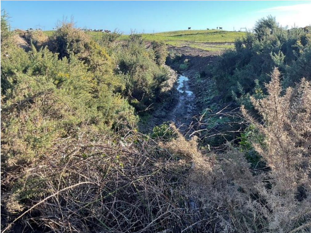
Photo 4. The created drain with excavated channel and banks.
