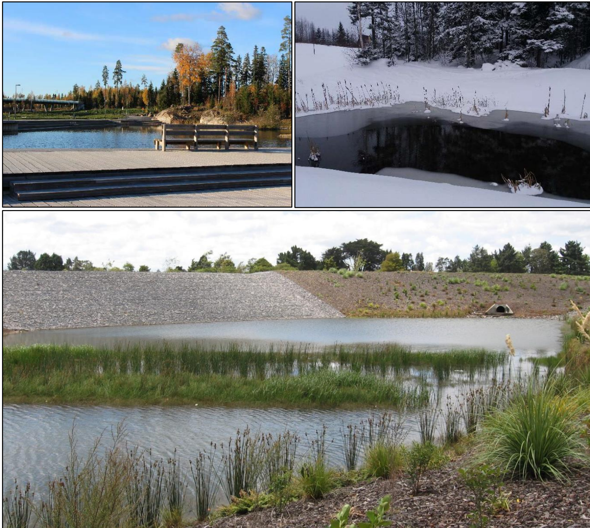
Figure 2-3: Wet retention ponds in Tampere, Finland (top) (pictures from Eisenberg and Polcher (2019)) and Auckland (lower). (picture from Dr Annette Semadeni-Davies).
