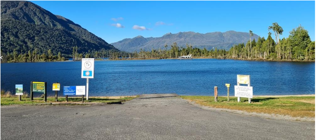
Figure 9 Lake Brunner Iveagh Bay boat ramp site
