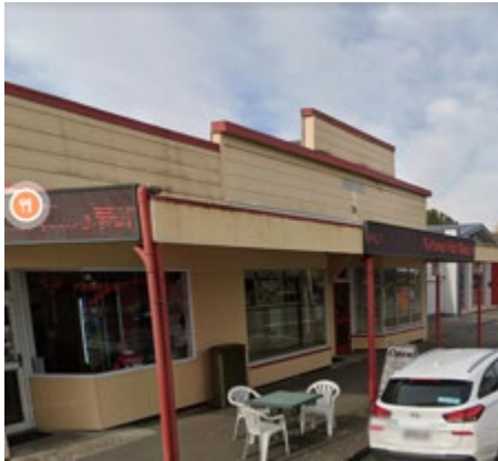
Roofline hidden behind parapet
