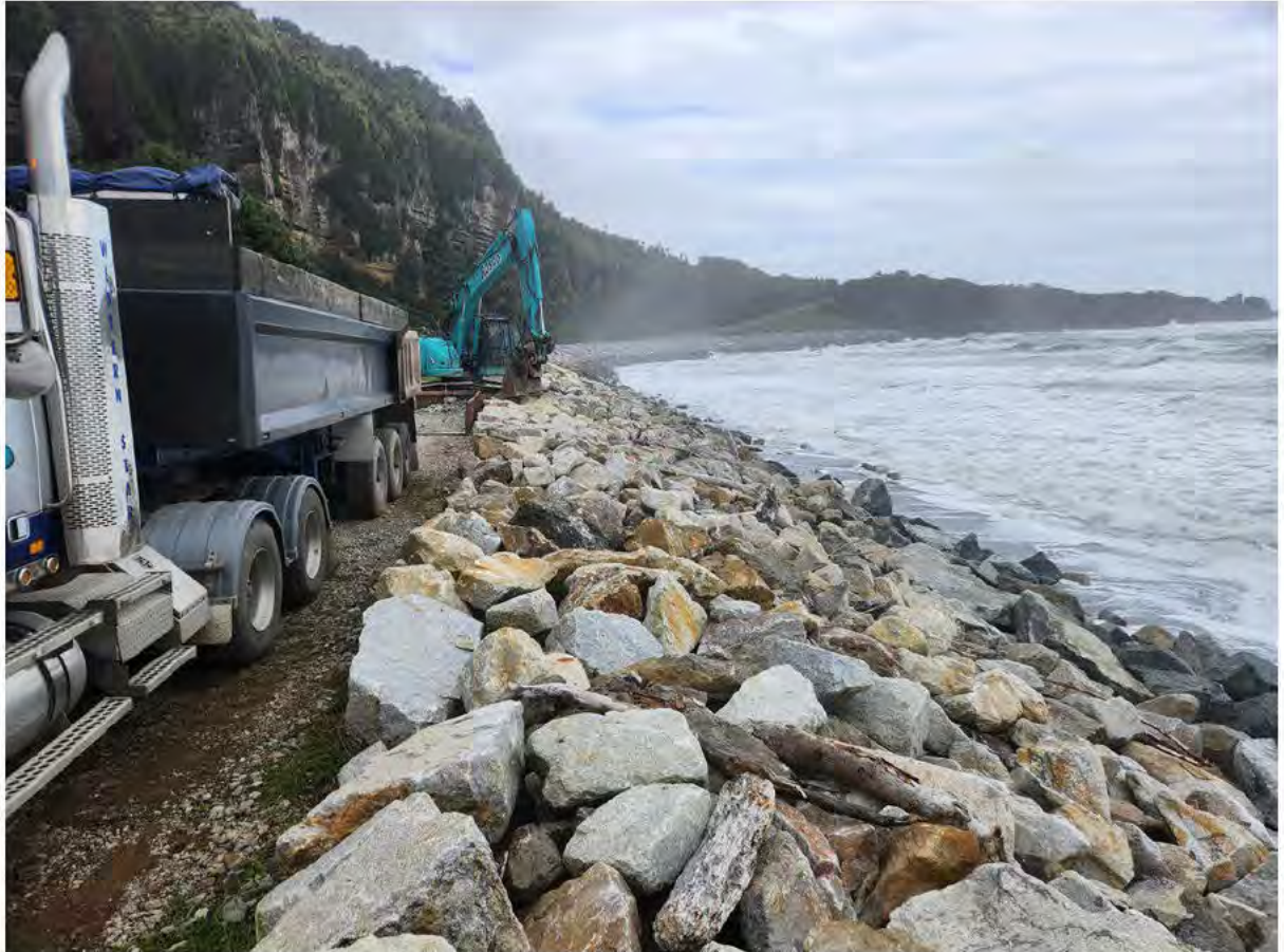
Image 1: [REDACTED] undertaking crest top up work (September 2023)
