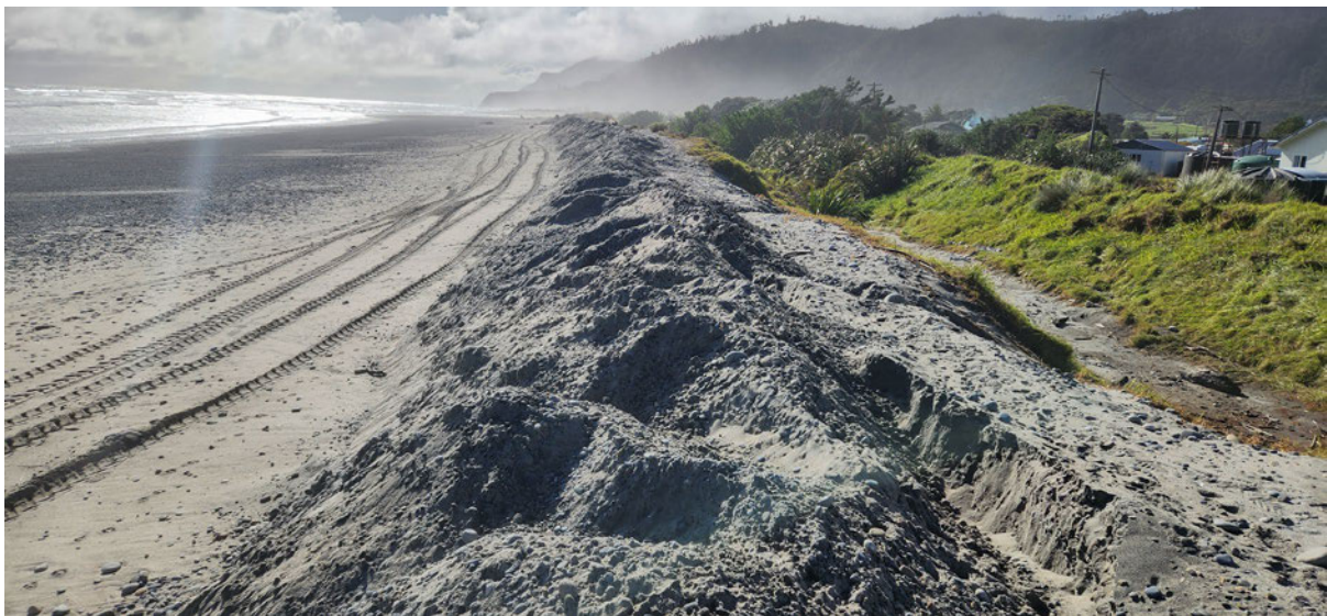
Figure 1: Sacrificial seawall post repair August 2023
