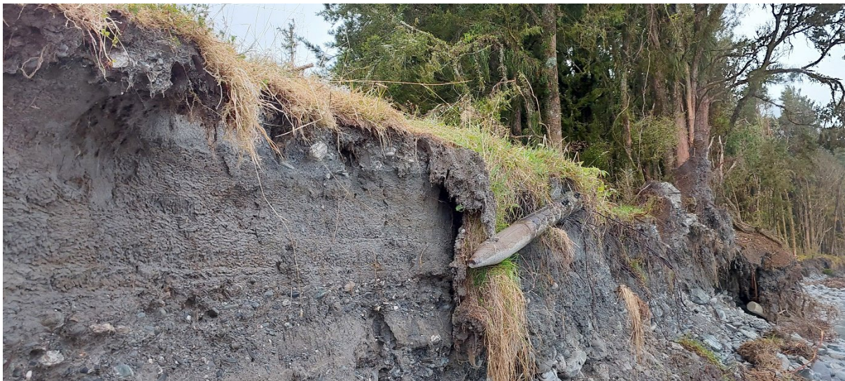
Figure 2: Bank erosion including compromised fencing
