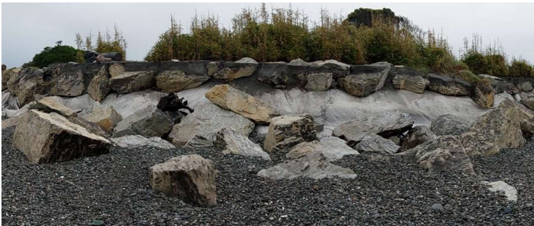
Figure 2: Boulders dangerously perched at the top of the slope shoulder.
