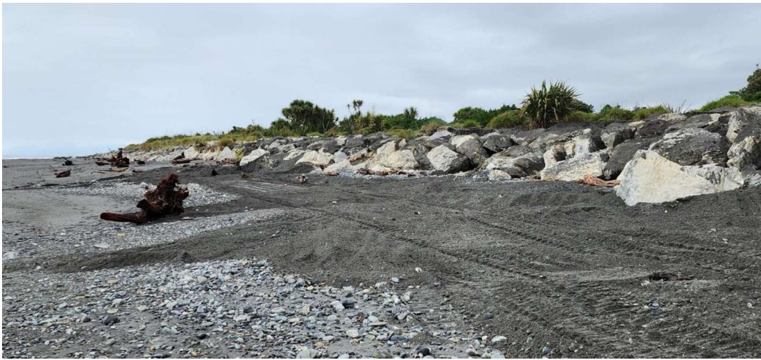
Figure 6: Completed work (northern section)
