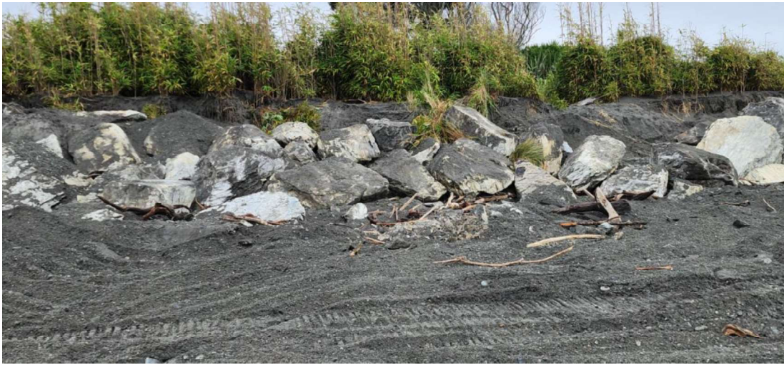
Figure 5: Completed work (same location as Figure 2)
