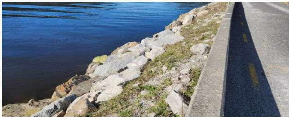
Photo 7: Placed rock riprap
