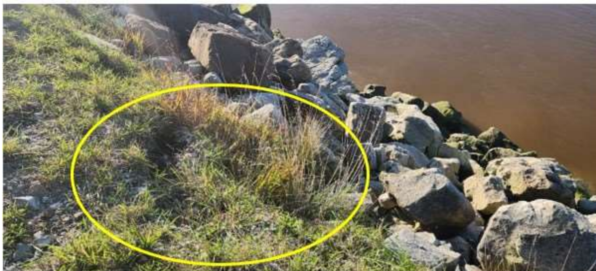
Photo 1: Slumped area
