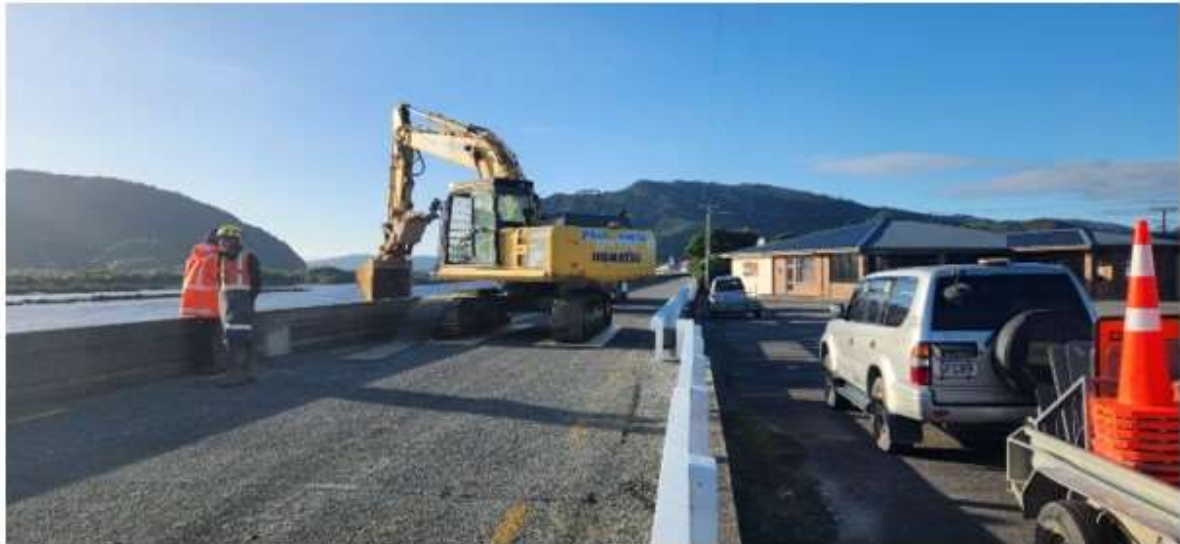
Photo 5: Placing rock using thumb.
