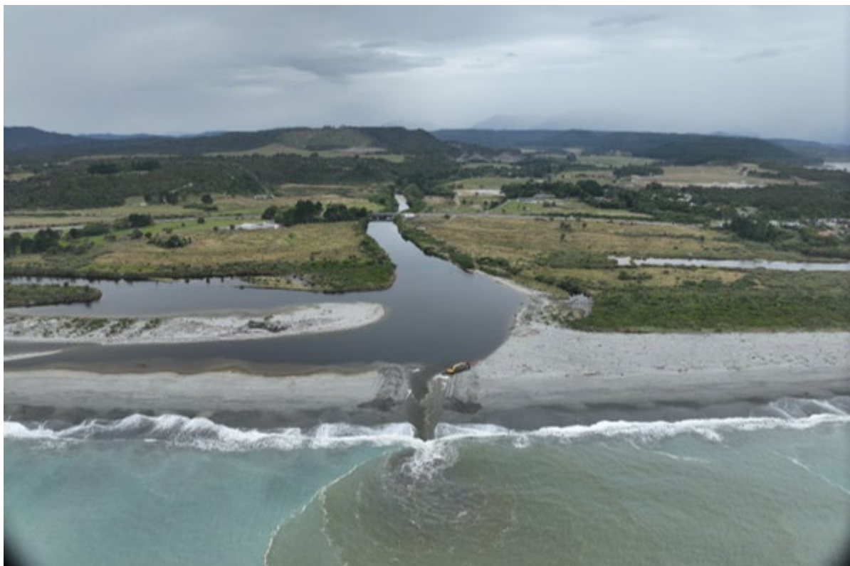
Figure 4 – Looking towards the New River Bridge and main road.
