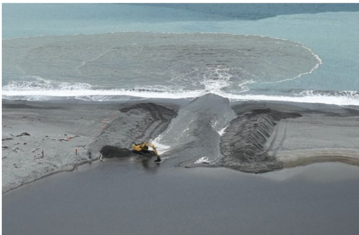
Figure 3 – Excavating the riverside plug of material
