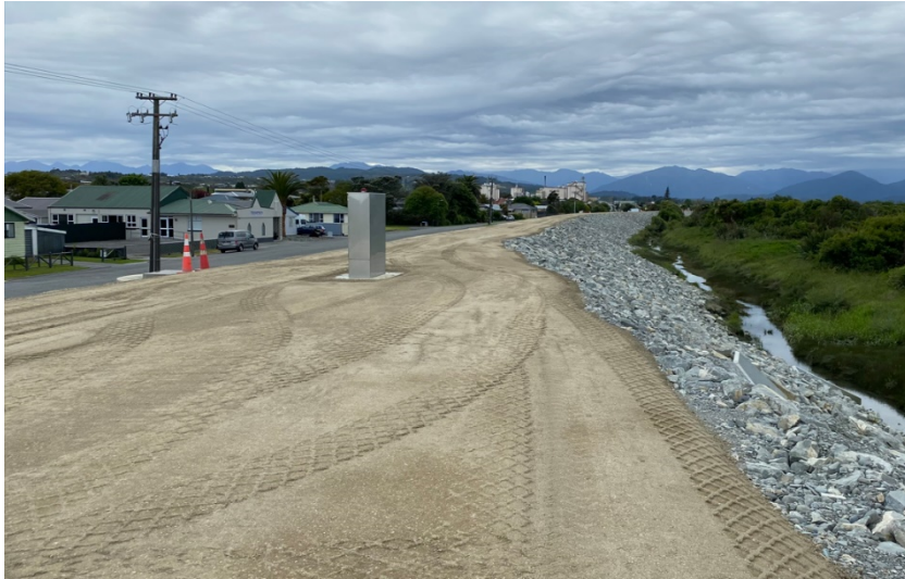
Cycleway surfacing complete
