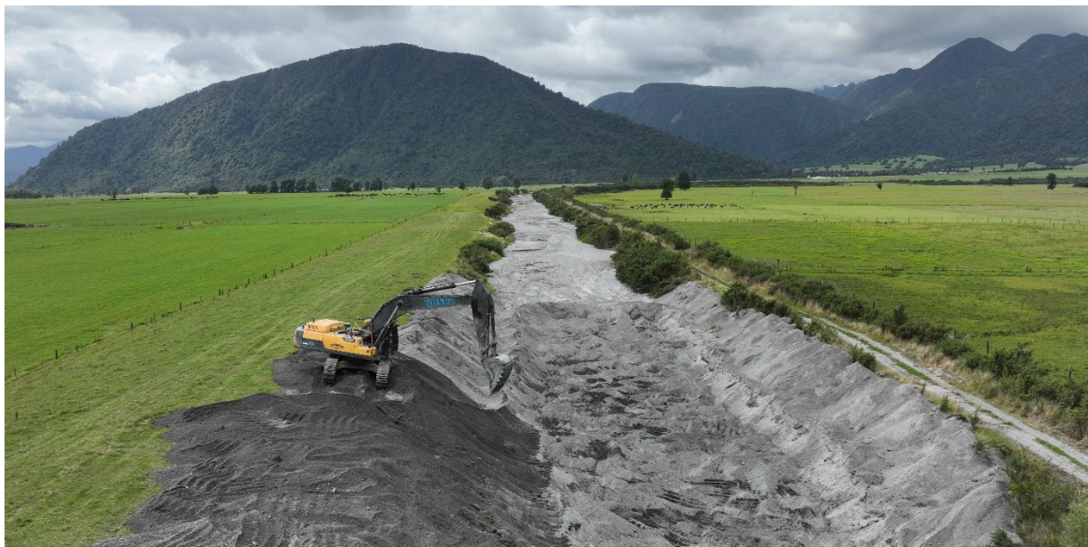
Figure 7: Clearing out of the riverbed in progress
