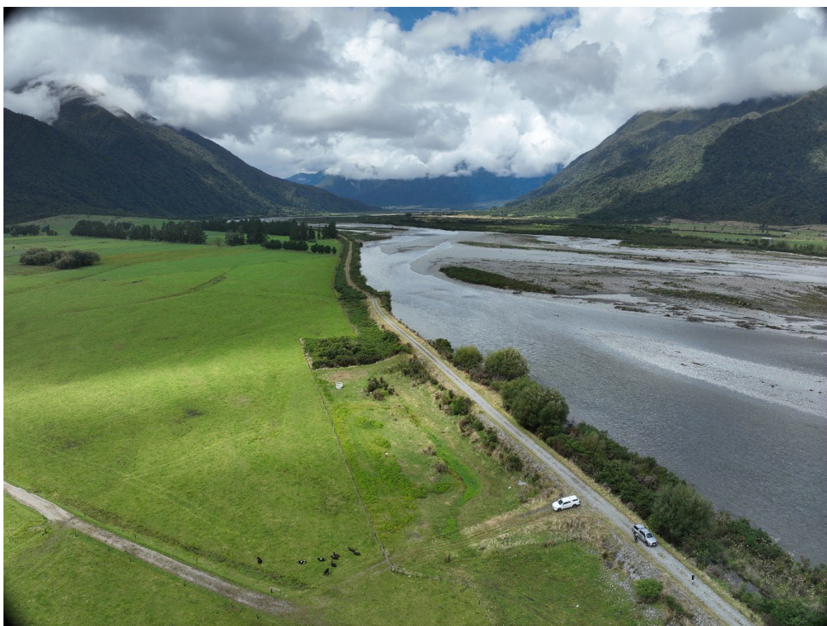
Figure 5 - Aerial view of the length of stopbank requiring top-up maintenance.
