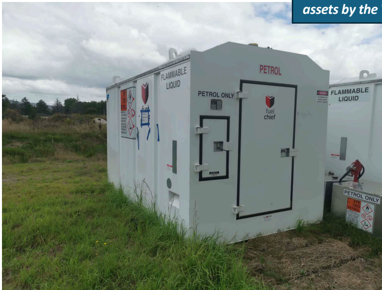
Figure 3 2x 15k, 1 x 5k amd 1x 2.5k litre tanks
