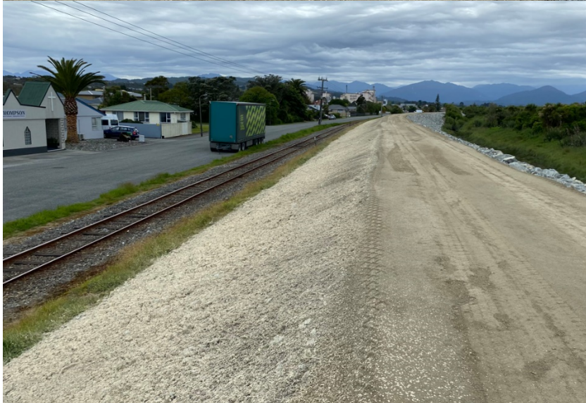
Hydroseeding complete, grass strike to be monitored
