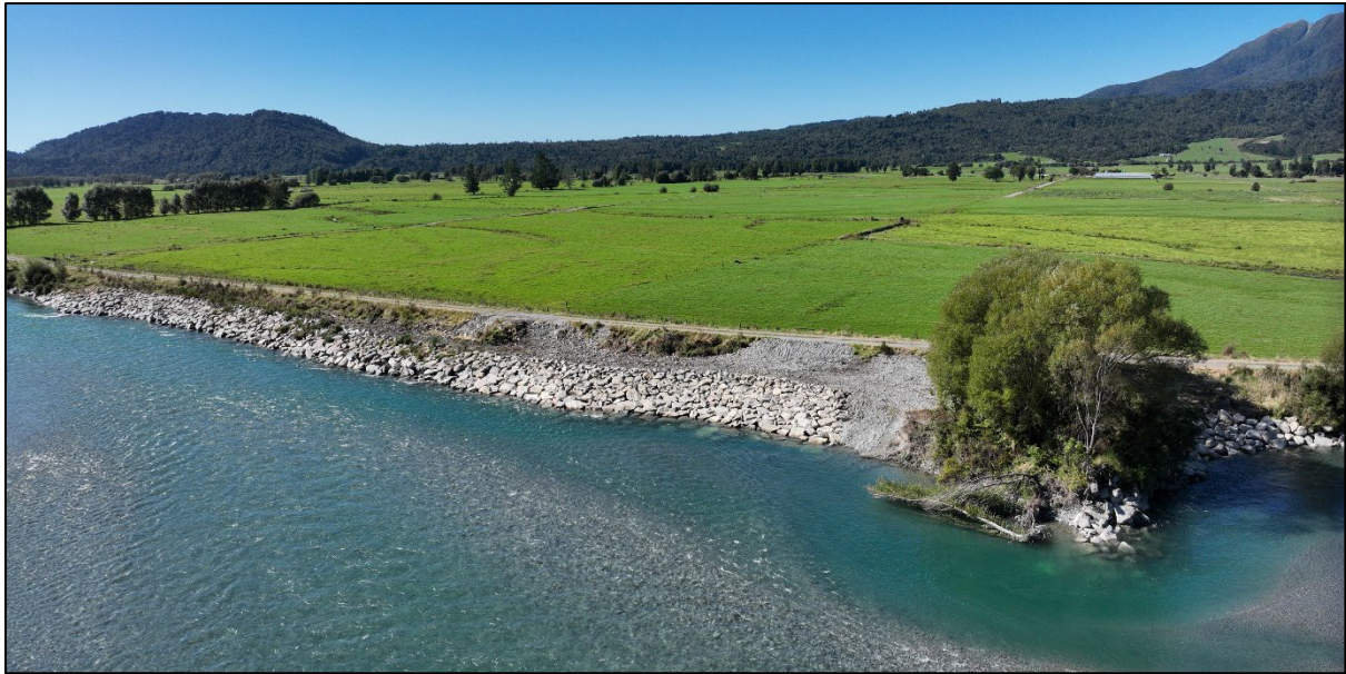
Figure 4: Taramakau post rip-rap repair on 20 March 2025.
