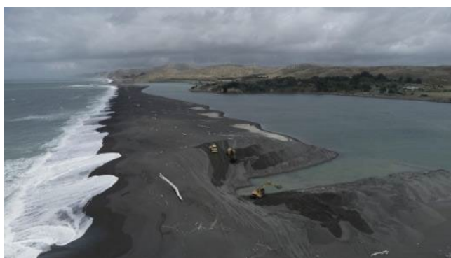
The position of the Wairoa River has been shifting west since 2016, reducing the efficiency of the river mouth. Image: HBRC
