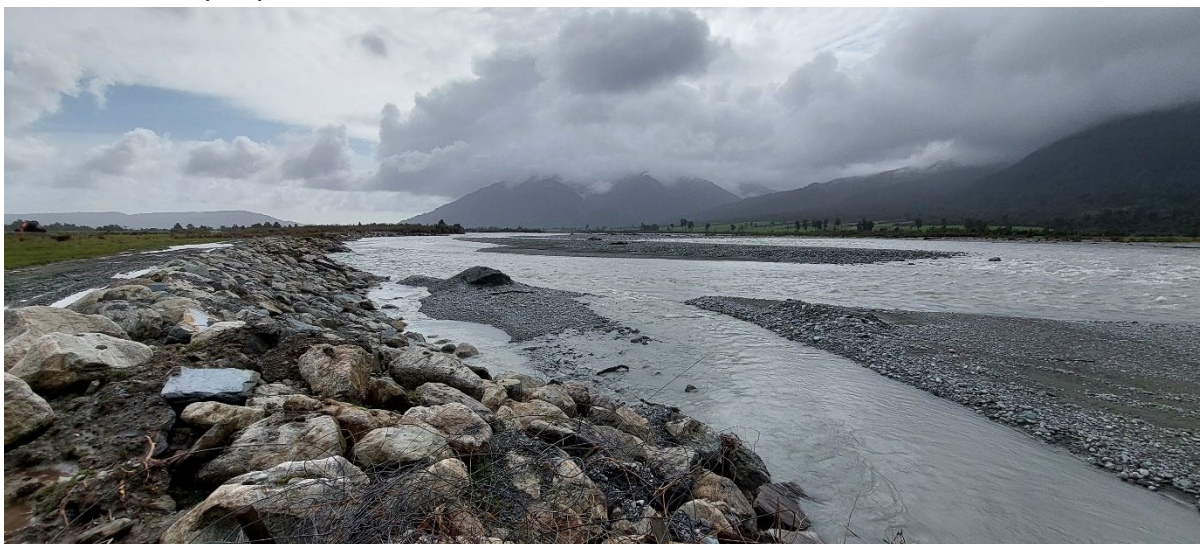
Figure 6: Post 400T placement
