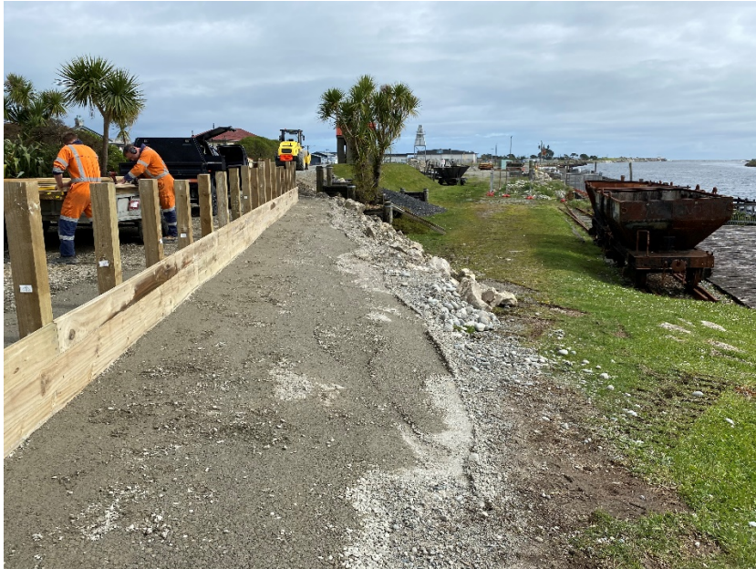
18 September 2024 Retaining wall to connect to Mawhera Quay wall underway
