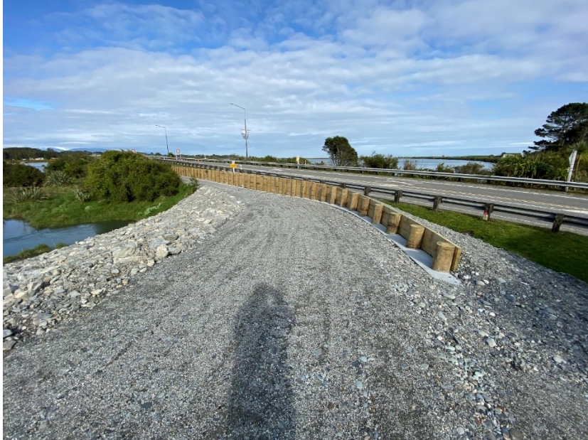
18 September 2024 Retaining wall adjacent to SH6 bridge complete
