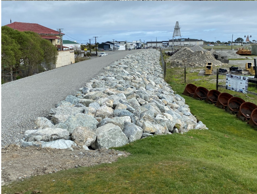
18 September 2024 Rock armouring along Gresson Street River frontage complete
