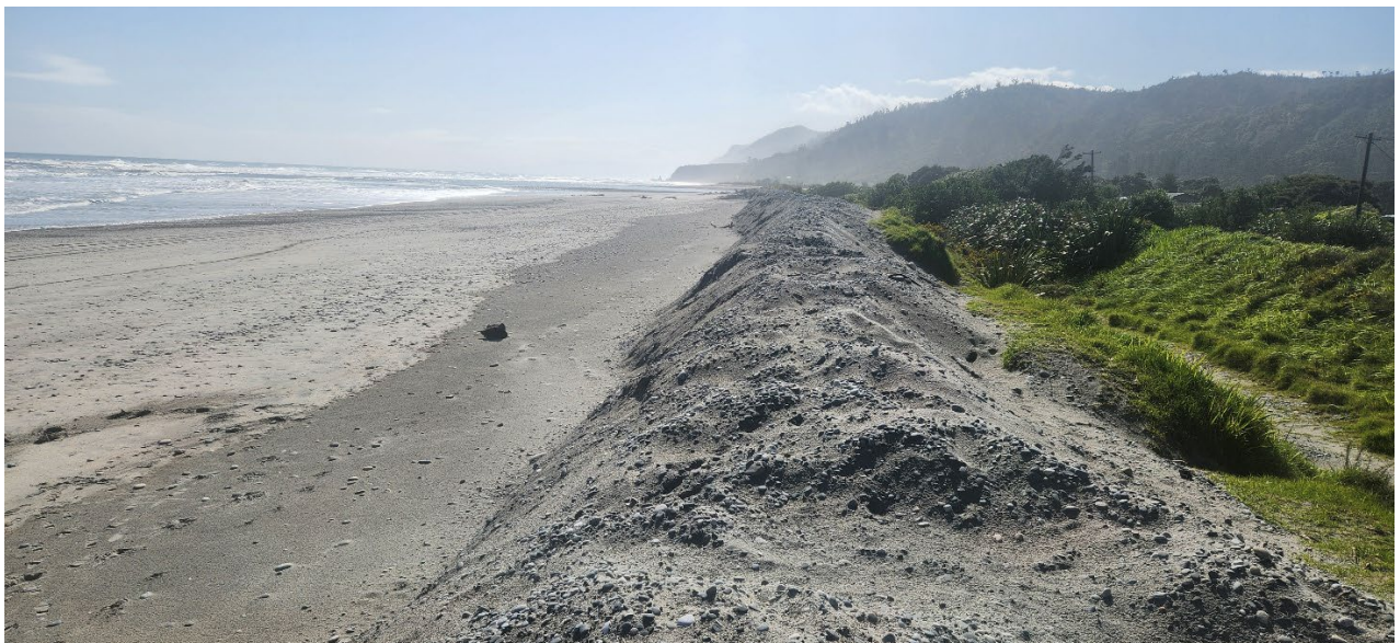
Figure 1: Topped-up sacrificial bund at Mokihiui
