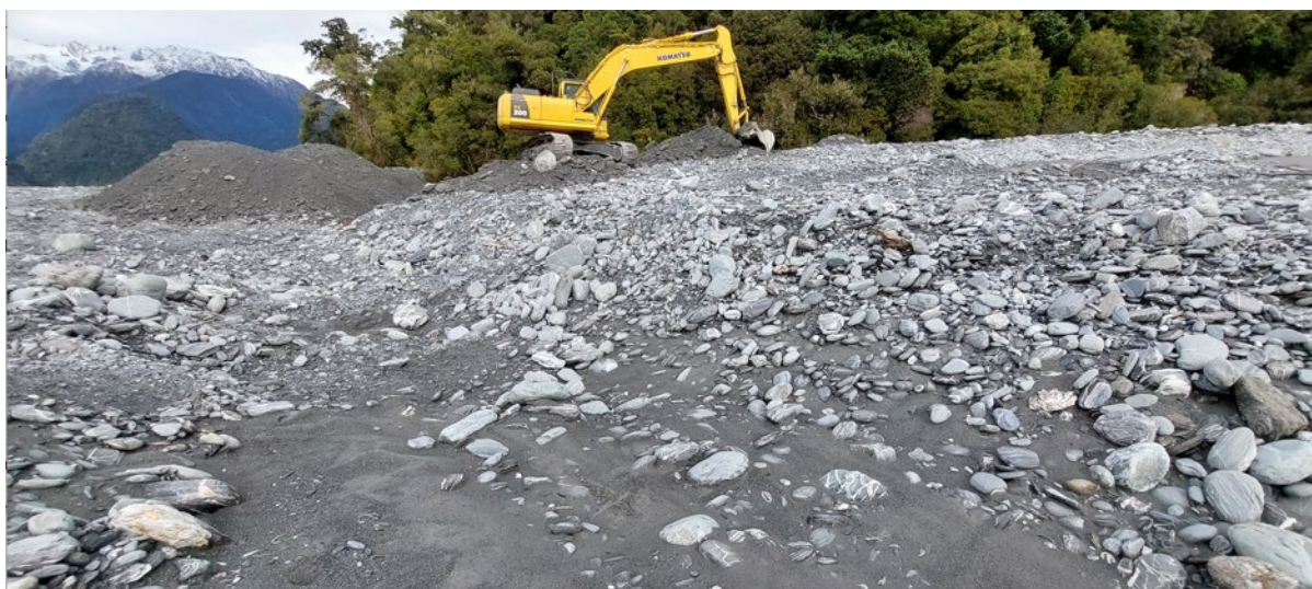
Figure 6: Preparations underway for spur reconstruction
