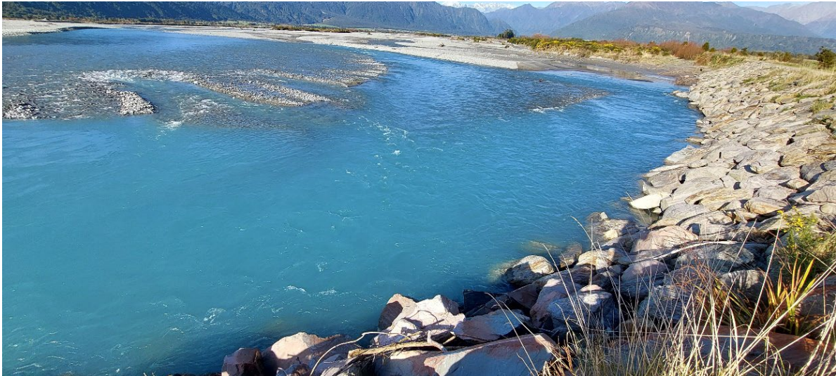
Figure 3: Henry Adams repair site
