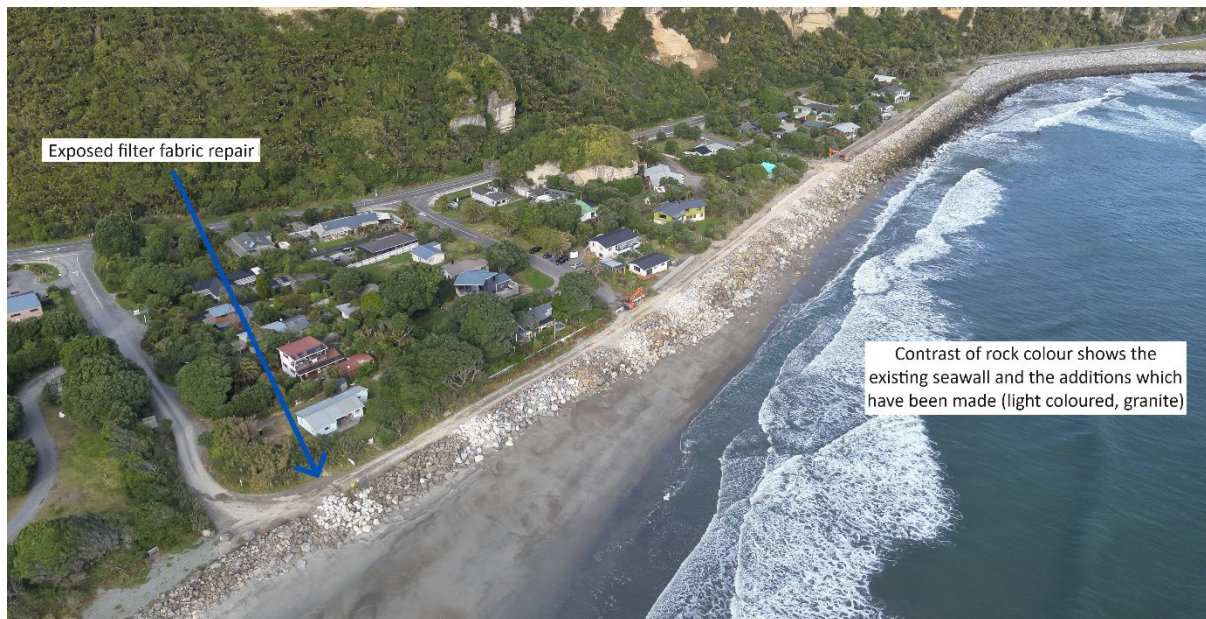
Figure 2: Punakaiki seawall repair work
