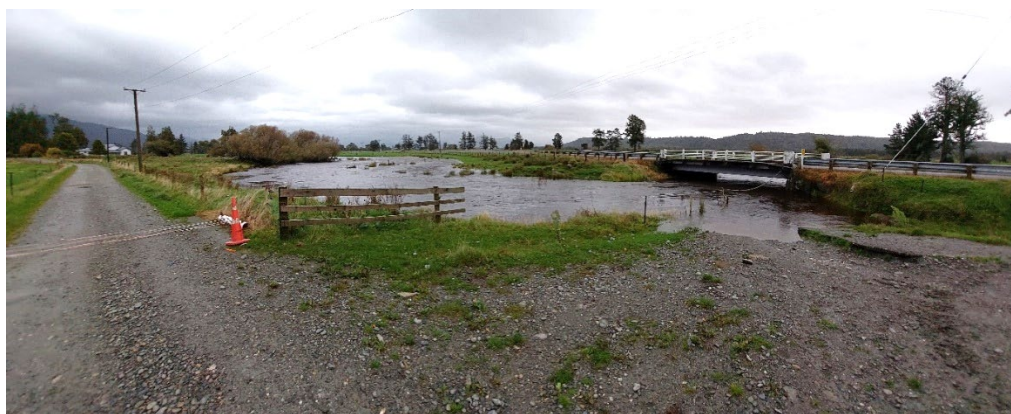
Figure 1: Raft Creek bridge
