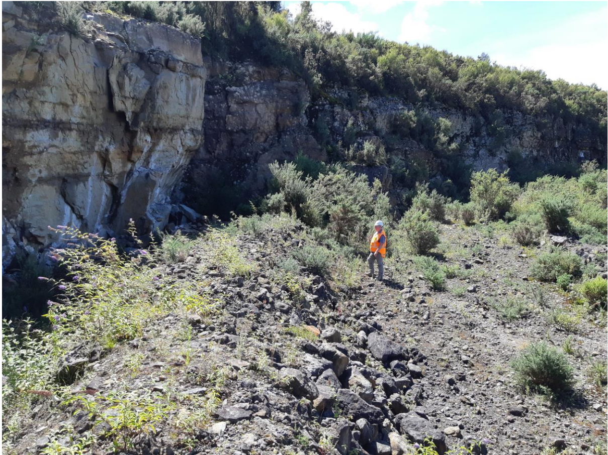
Site Photo 15 Western pit wall. A bund has been constructed at the toe, refer to Site Photo 14 .
