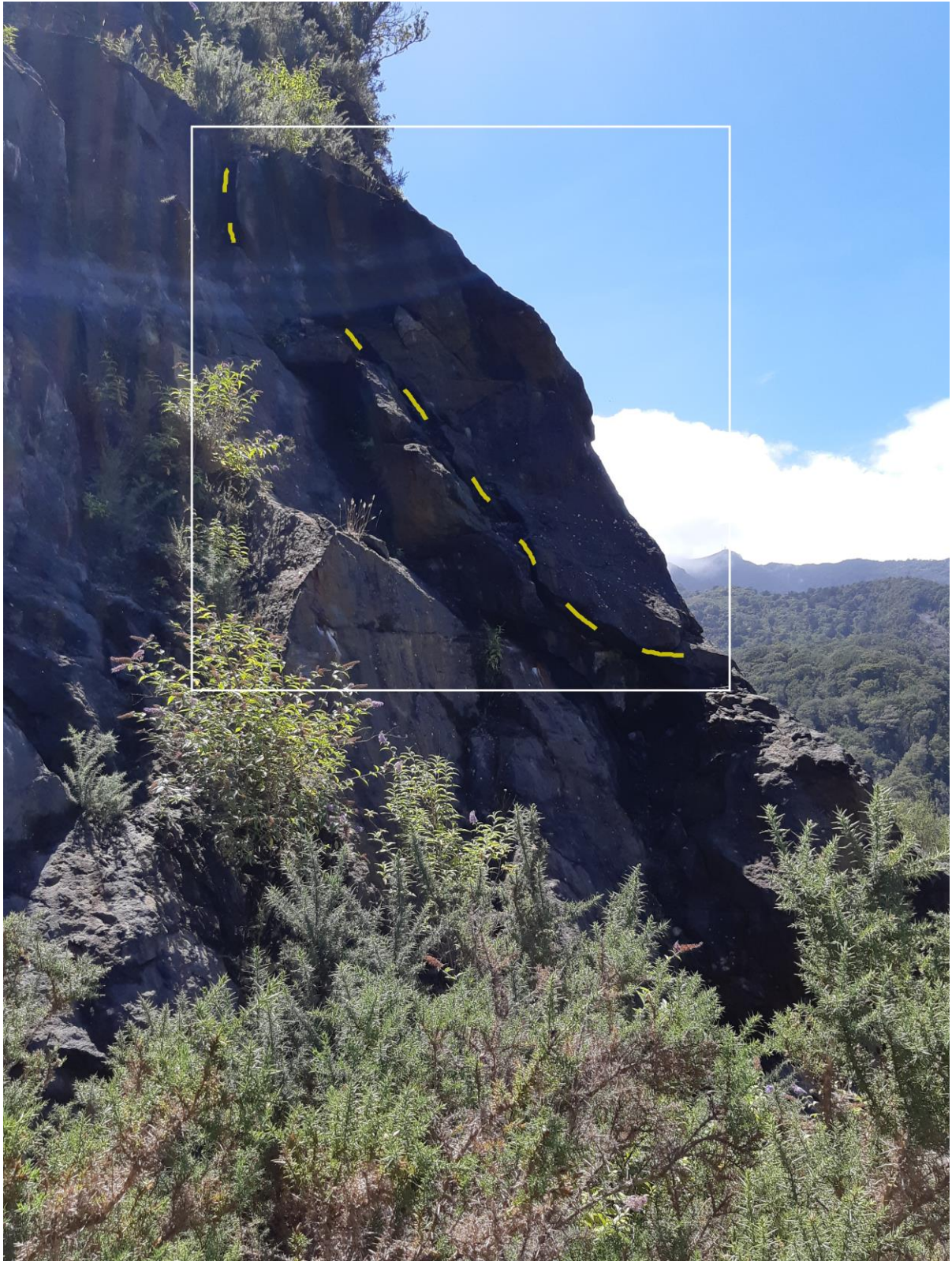
Site Photo 13 Lower batter of the Nose. Large slab (estimated at 3x2x1m) of rock appears to be partly detached.
