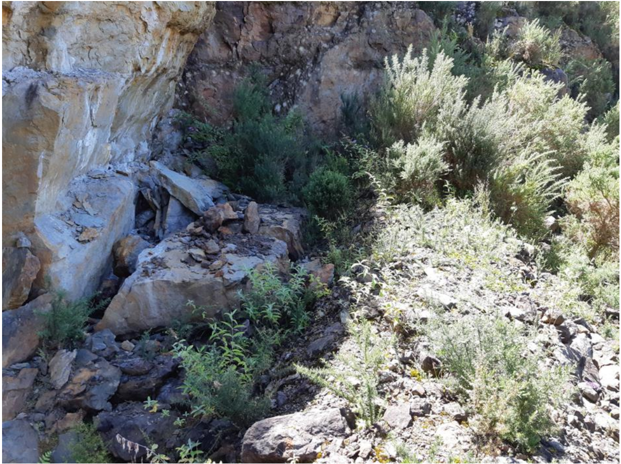
Site Photo 16 Western pit wall. Large block of sandstone caught behind earth bund (post 2015 rockfall).
