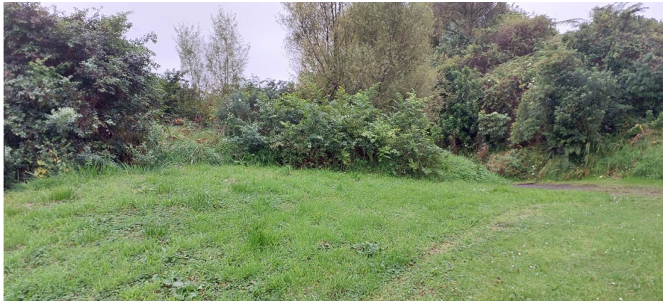
Figure 3: Vegetation maintenance required on asset
