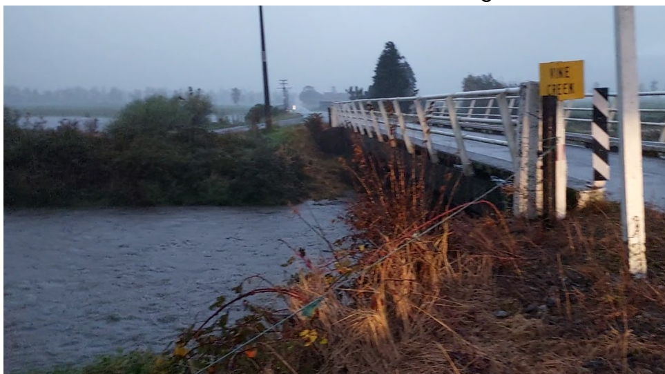
Figure 2: Vine Creek bridge
