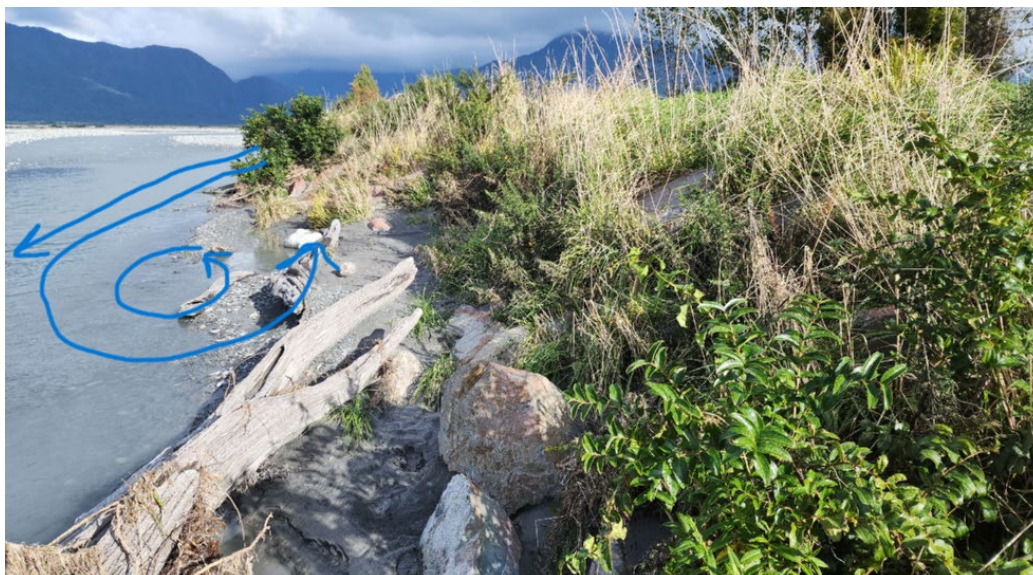
Location: Left bank, an eddy has caused minor erosion behind a spur that will need ongoing monitoring.
