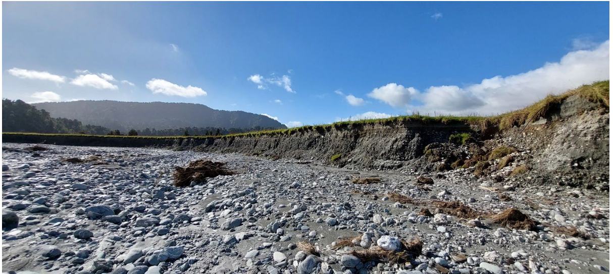
Figure 5: significant erosion down stream of Havills wall
