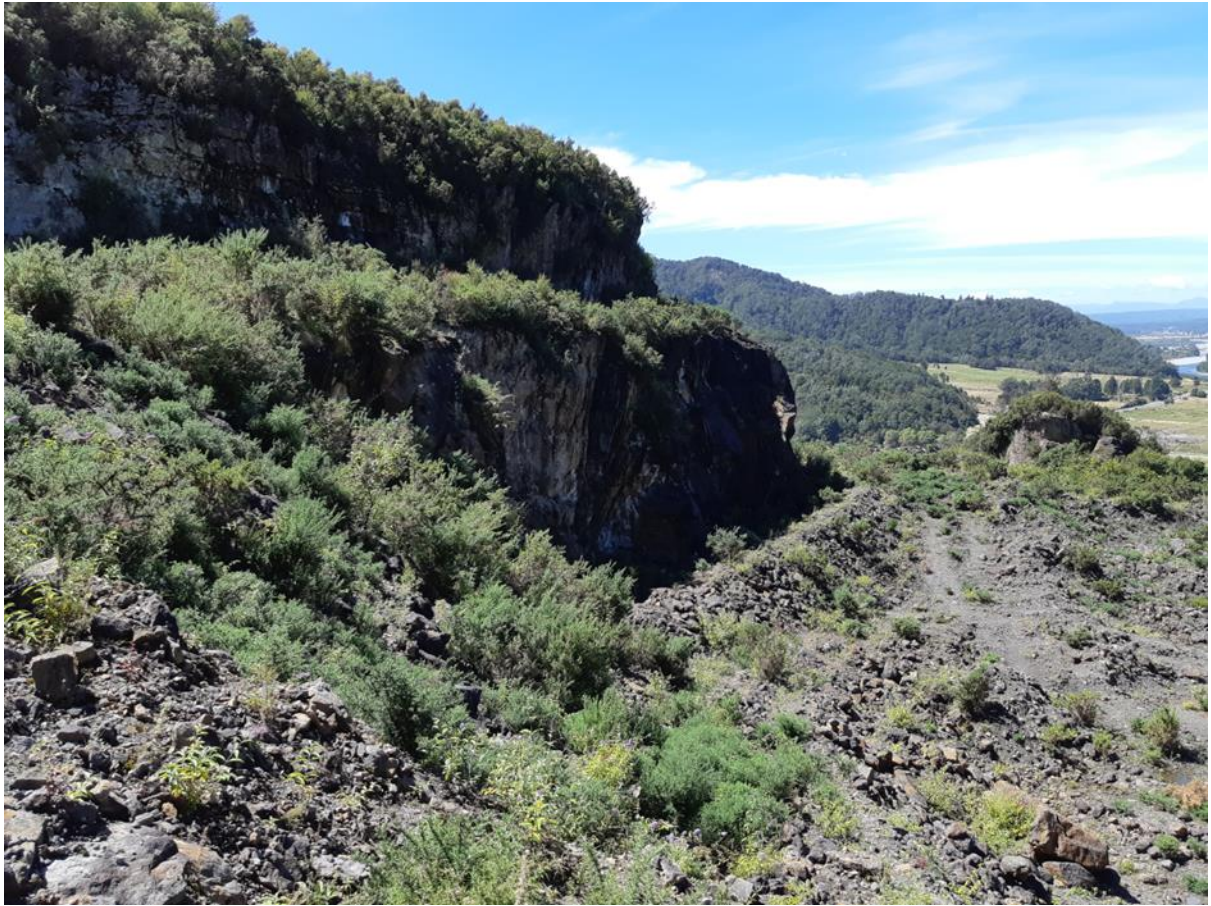
Site Photo 14 Northern highwall, looking east.
