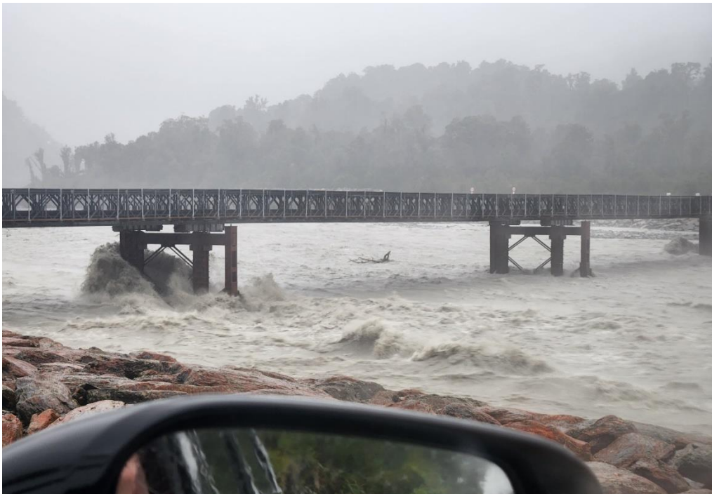
Looking upstream at the State Highway Waiho River bridge piers
