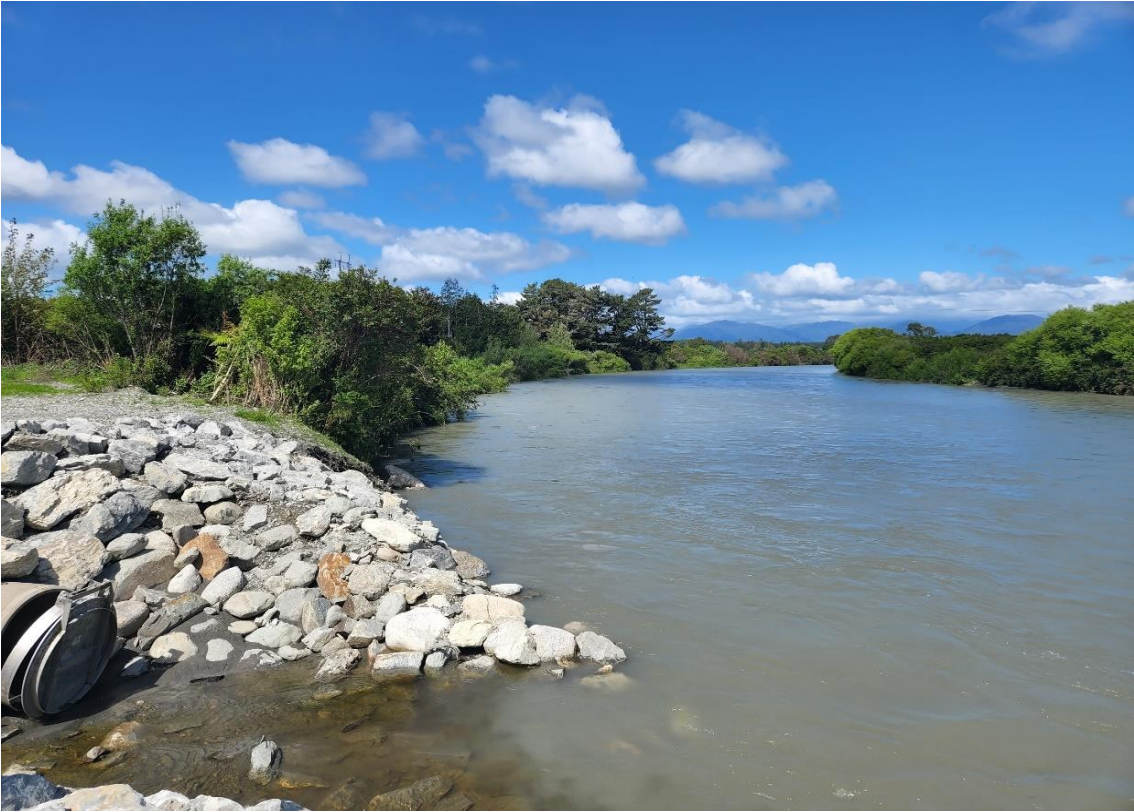
Looking upstream at the true left bank 04/11/2022
