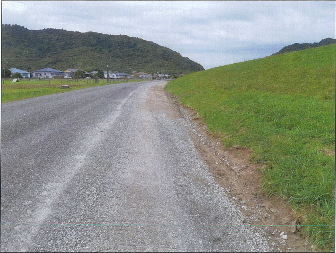
Stopbank toe at completion of drainage improvement works
