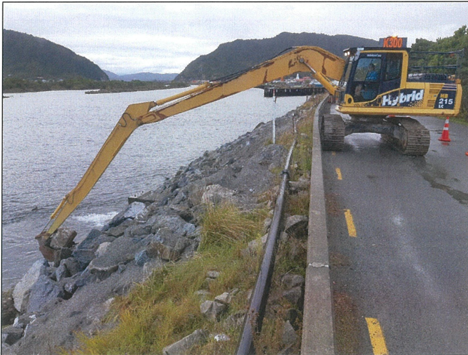
Long-reach digger doing the final placement of the rock.
