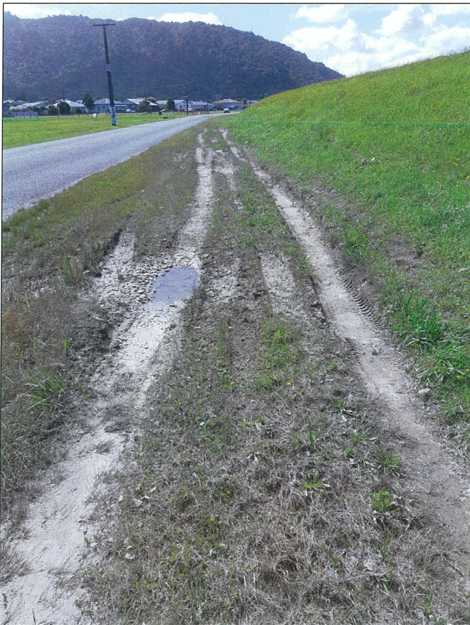
Before drainage works
