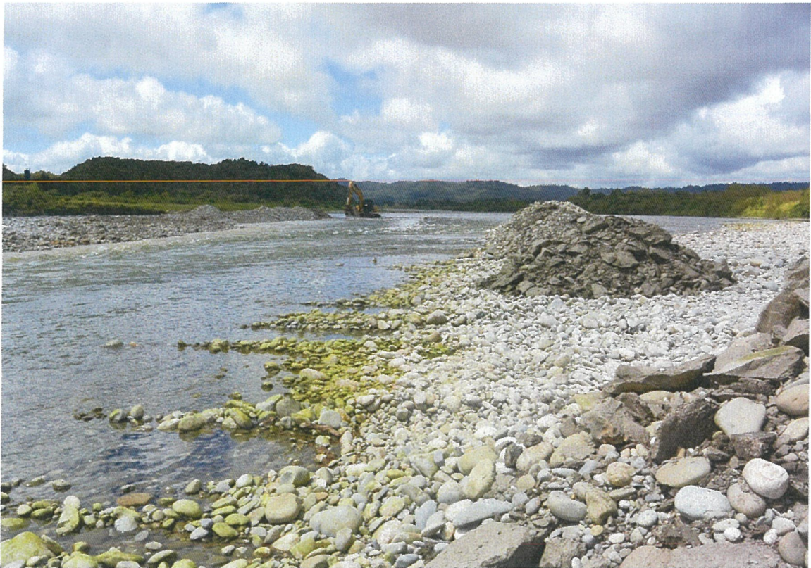
Looking upstream along the diversion cut
