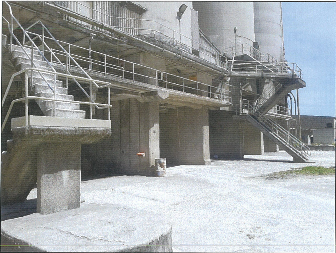
Example of concrete structures to be demolished
