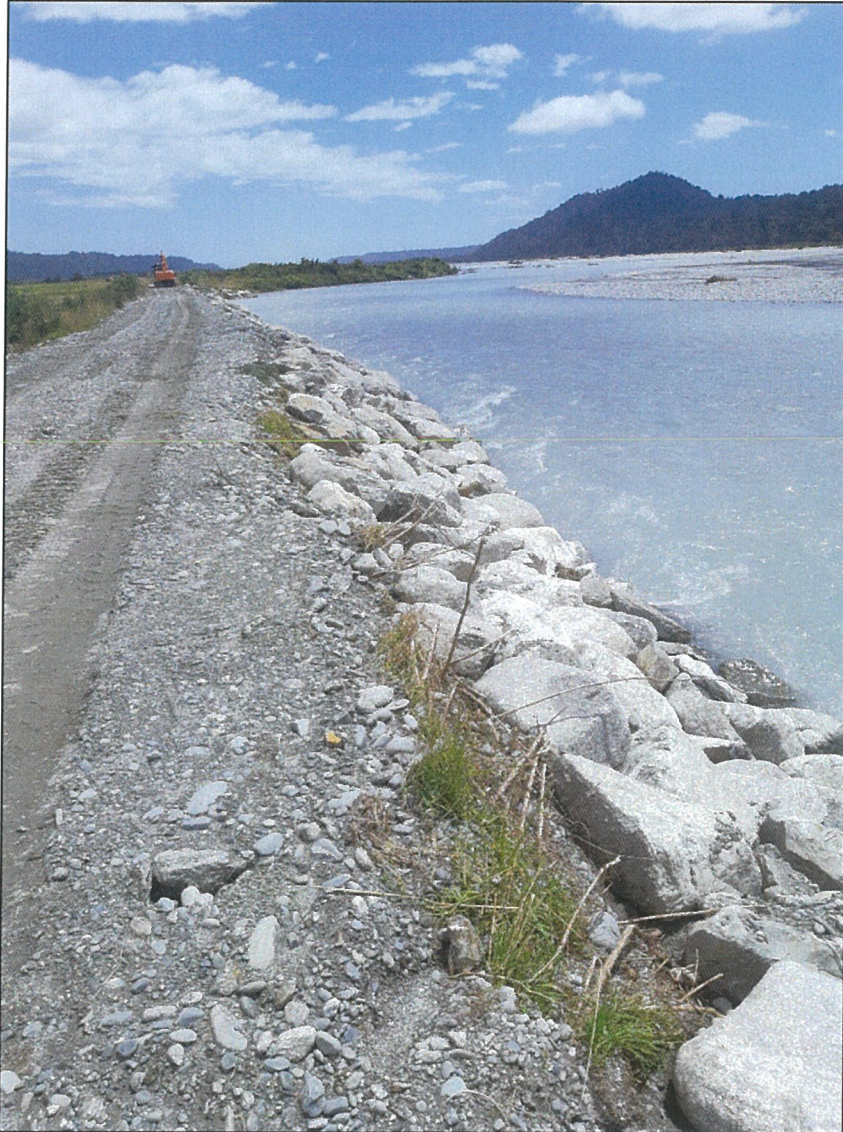
Completed Rock Rip Rap
