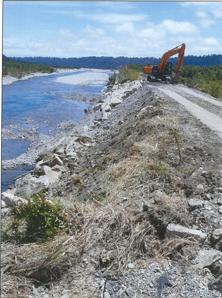
Rock Riprap being installed
