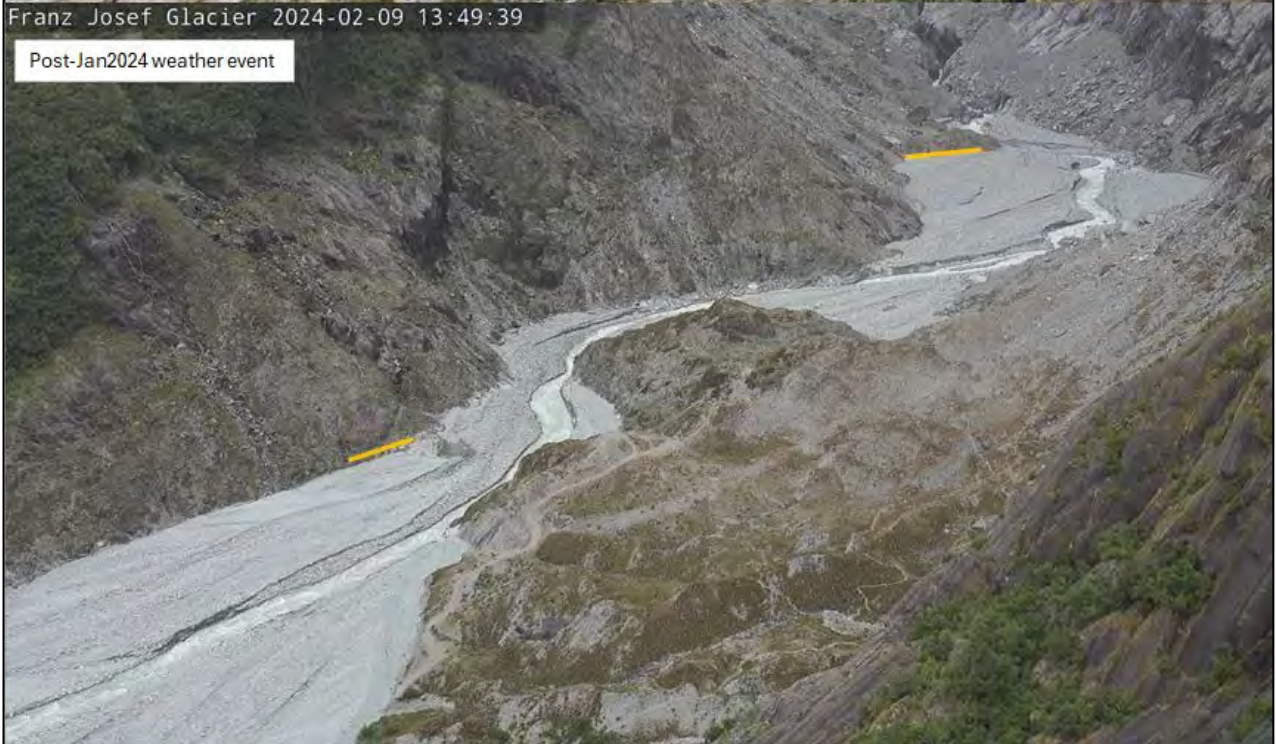
Figure 4-10 – Fixed camera 6 images from before and after the January 2024 event. The orange lines have been added for reference.
